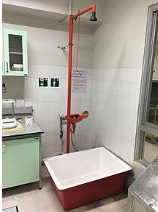
Emergency eyewash and shower – Image by Korn966 is licensed under CC BY-SA 4.0 Meters
